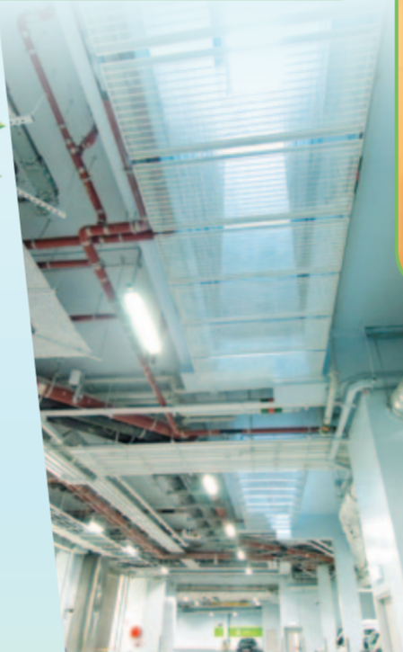
地庫停車場太陽能煙囪系統通風口 Solar chimney ventilation opening in the basement car park
