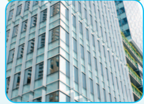
縱向和橫向遮擋太陽裝置 Vertical and horizontal sunshades
